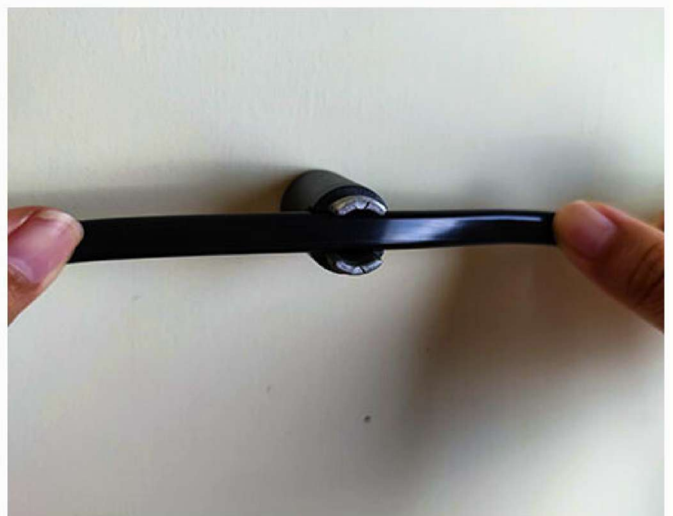
② Fix the cable to the holders
